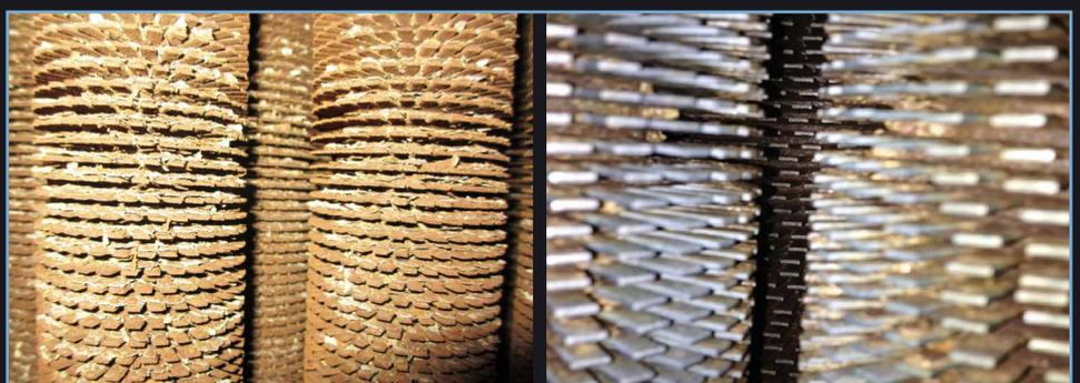
HRSG FIN TUBES BEFORE AND AFTER DRY ICE BLASTING
